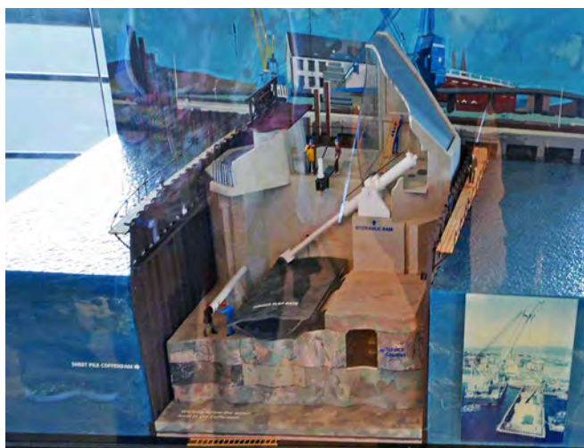
Cross section of the Weir showing the huge hydraulic rams that lift the flap gates, the service Gallery tunnel crossing the river bed below, the sheet pile coffer dams used to hold back the water during construction of the Pier Houses, and the 30m long steel tube piles used to punch through the Belfast 'sleech' (a soft mixture of sand, gravel and boulder clay) to the firm sandstone bedrock below
